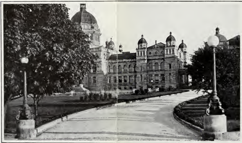
Hassam Pavement in Driveway, Parliament Building Grounds, Victoria, British Columbia
